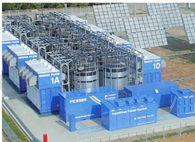
Figure 2. 2MW/8MWh VRFB demonstration system at Yokohama, Japan. Picture from [7].
